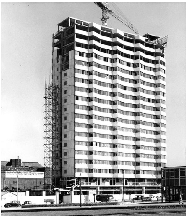
Arlington House under construction
