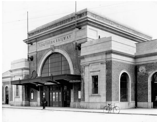
The old and new Margate Railway Station
